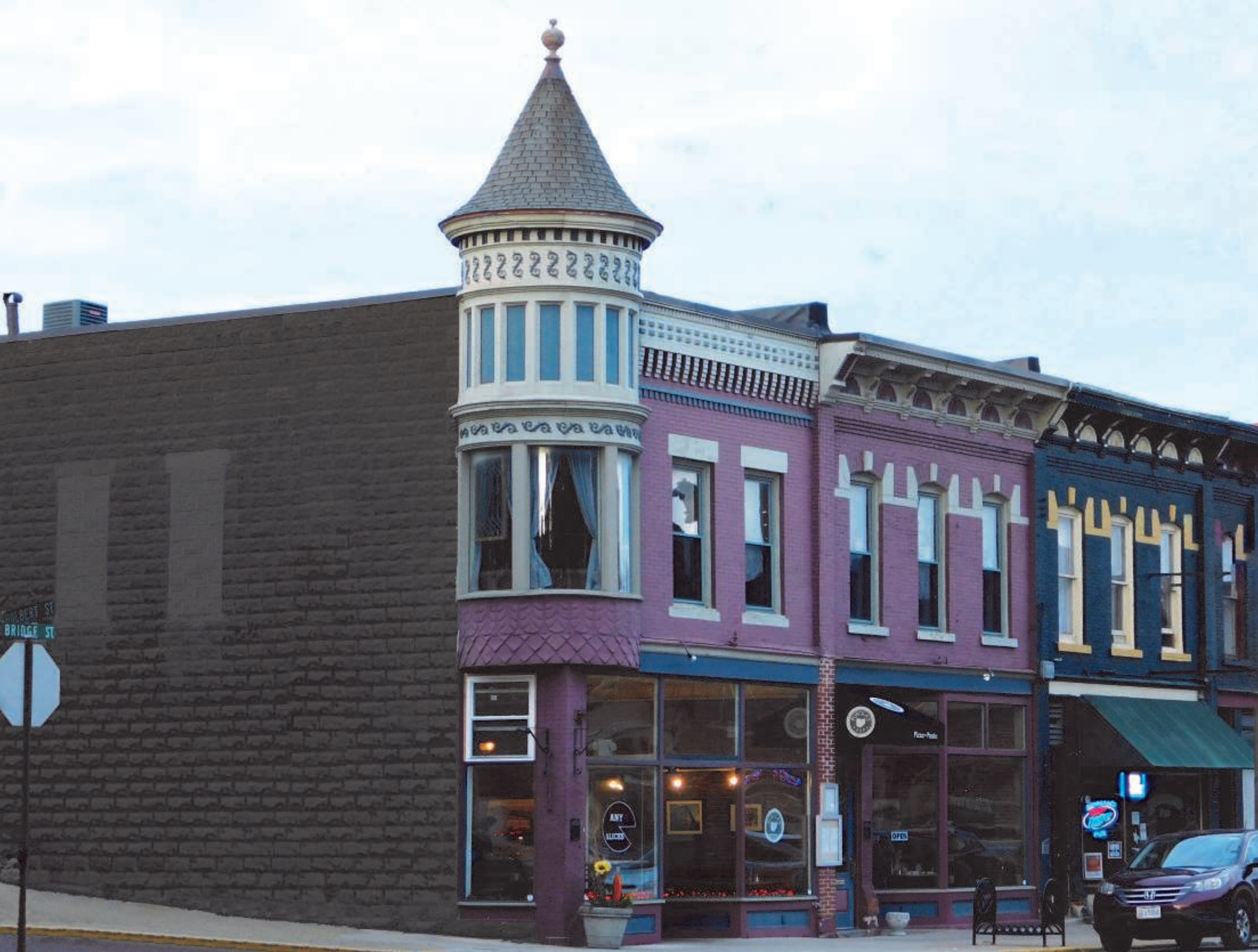
This Architectural icon located on Bridge Street in the Ashtabula Harbor was known for many years as Hulbert's Restaurant. In 2005 it was listed, marketed and SOLD by Walt Poff of Nova Star Real Estate to David Parsons and became known as the Bridge Street Bistro. David has since passed but the vision he had for the Harbor Area is still remembered. Photo Credit: Walt Poff
