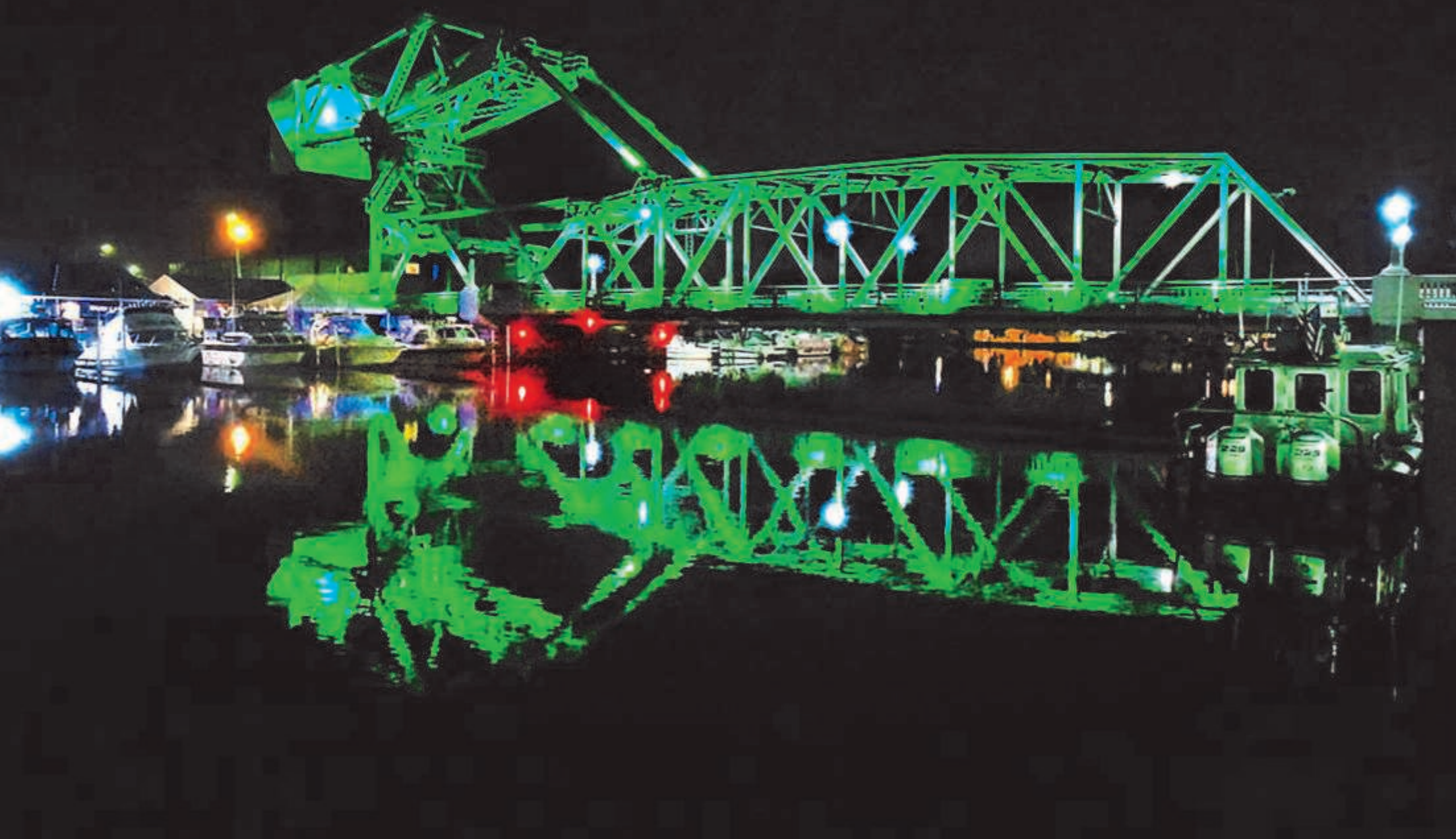
Built in 1925 by the Kelly-Atkinson Construction Company and the Fort Pitt Bridge Works on SR 531 spanning the Ashtabula River. The bridge is also known as the West 5 th Street Bridge and the Ashtabula County Lift Bridge. The bridge was listed on the National Register of Historic Places in 1985 as the West Fifth Street Bridge (NRHP # 85001801) The bridge was rehabilitated in 1987 and is a sight for visitors to see. Photo Credit: Dee Riley
